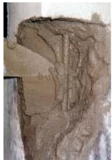
Apply the mortar
