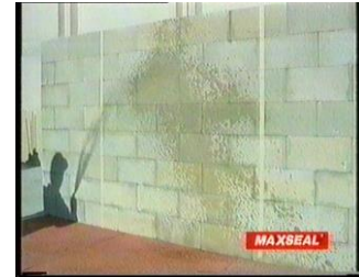
Wet surface before application.
