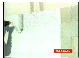
... finish using texture roller.
