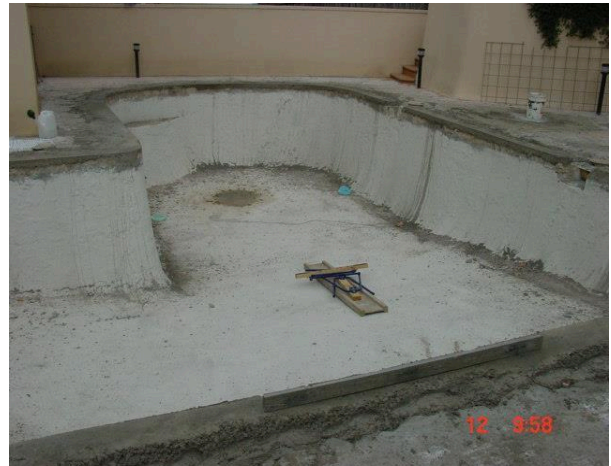
The bare concrete shell.
