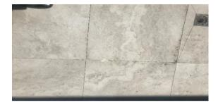
a. Remove all loose material as well as cleaning out missing grout areas – if efflorescence, apply Efflorescence Rid using Efflorescence-rid sprayed via a low-pressure sprayer.
