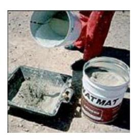
**Application:** Mix the required amount of WATMAT, place it around the perimeter of the hole, place the leveling tool on top and inside.
