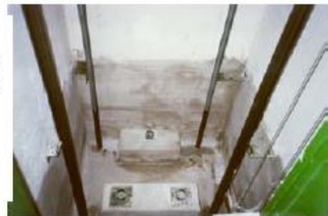
Lift Shaft full of water (left) and the same lift shaft after treated with DRIZORO MAXSEAL & MAXPLUG (right).
