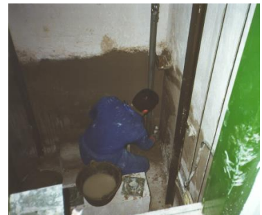
Applying MAXSEAL FLEX to seal the surface immediately after MAXPLUG (above).
