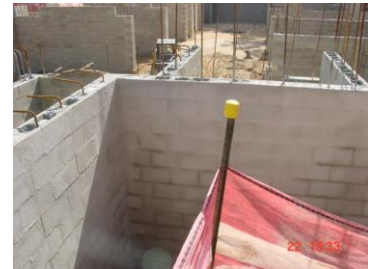
First coat finished.
