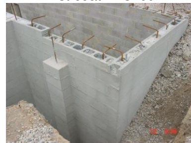
Second coat finished and partially backfilled.
