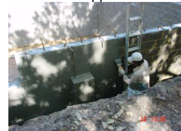
First coat of Maxseal Foundation.
