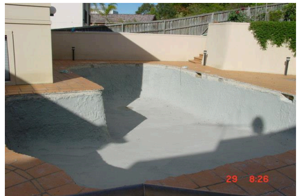
The pool after two coats of Maxseal Flex.
