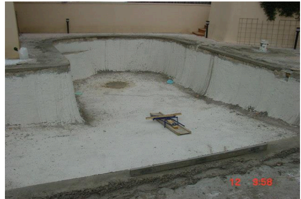
The bare concrete shell.
