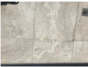
a. Remove all loose material and efflorescence as well as cleaning out missing grout areas – apply Efflorescence Rid using Efflorescence-rid sprayed via a low-pressure sprayer.
