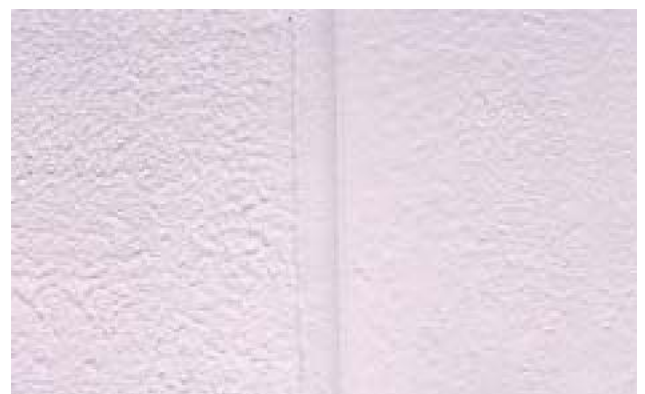
View of the finish joint. It can be painted with the desired colour.
