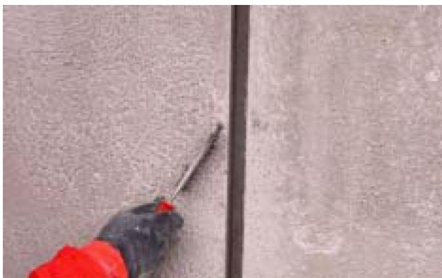
Preparation and cleaning of joint
