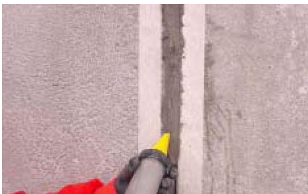
Application of MAXJOINT® ELASTIC
