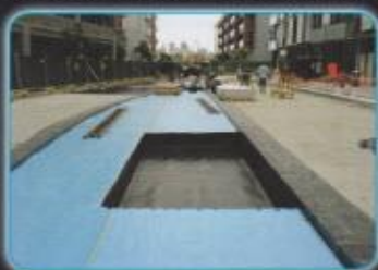
External Protection of Membranes Prior to Backfilling & Landscaping
