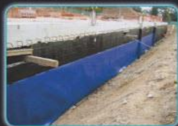
External Protection of Membranes Prior to Backfilling & Landscaping
